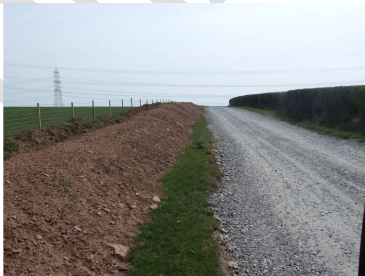
Access to working area. Topsoil is stripped to one side before stone is laid on geotextile membrane. Area is fenced off with stock-proof fencing or post and rope.
