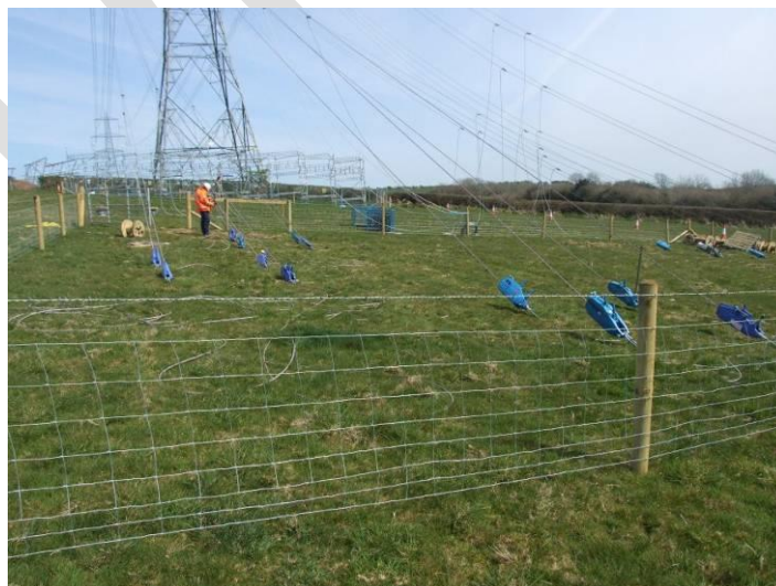
Ground Anchors (buried)
