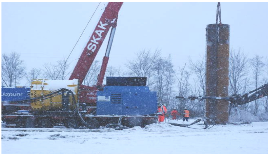
Figure 1 Pile crane and gripper (left) with pile hammer (right)
