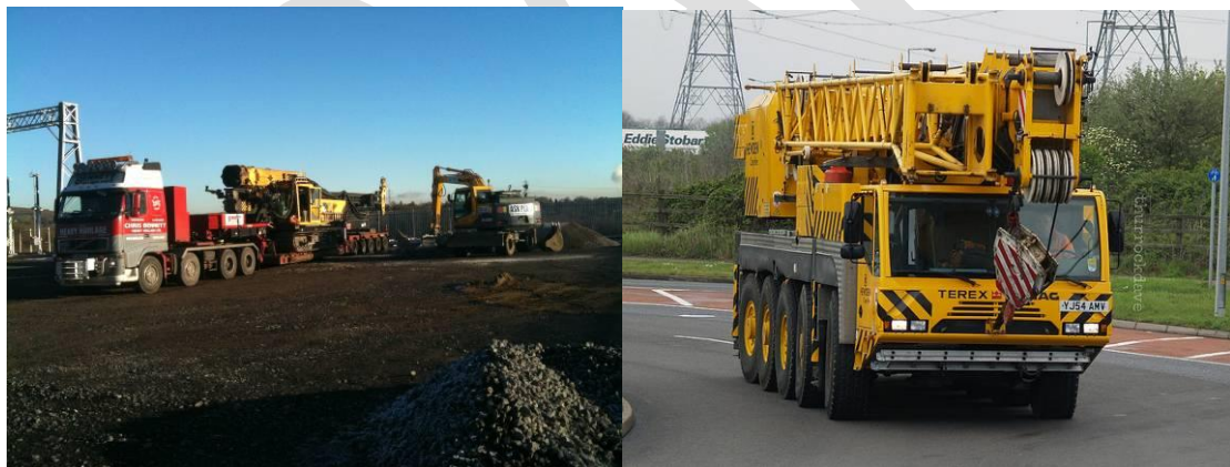
Access will be required for large vehicles during construction
