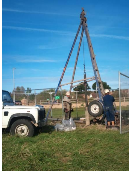
Set-up of a typical percussive borehole rig
