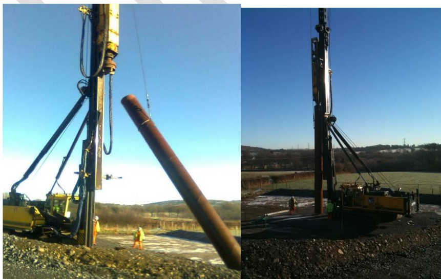
Piles being lifted into position to be driven into the ground.
