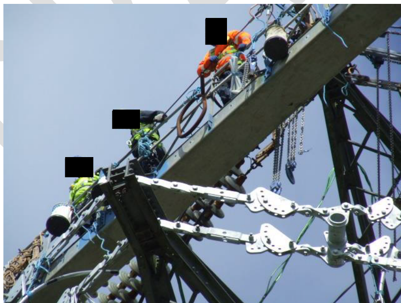
View of men working on a pull through pylon and access platform
