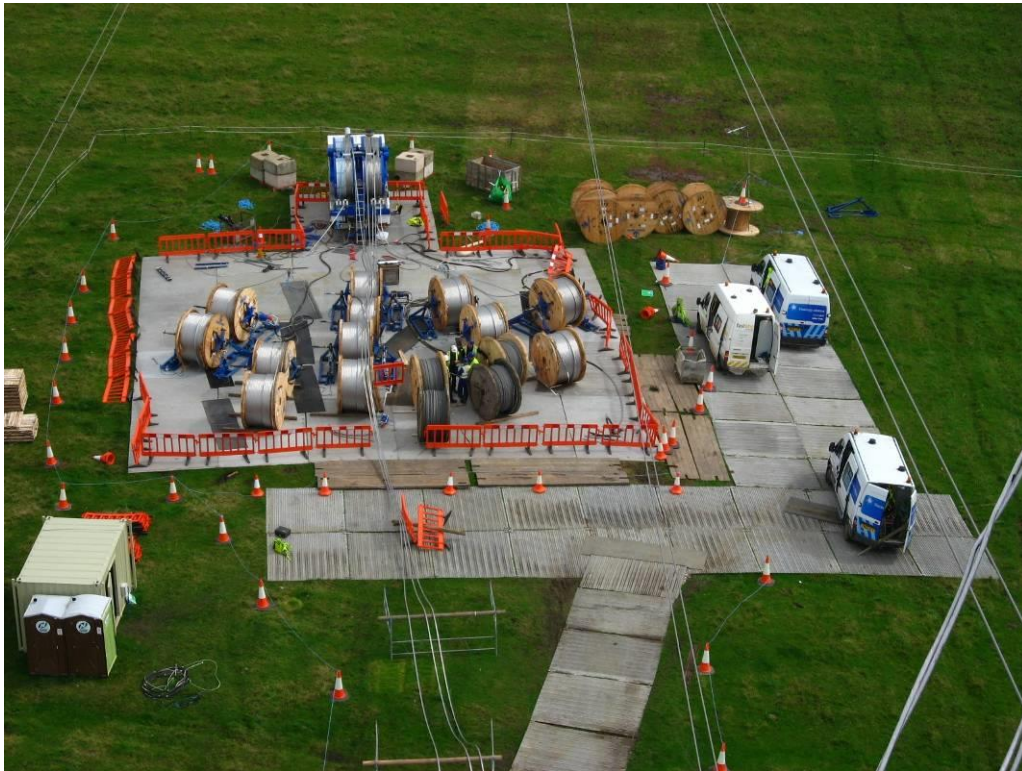
Typical Machine sites on EPZ, with tensioner machine and new conductor drums.
