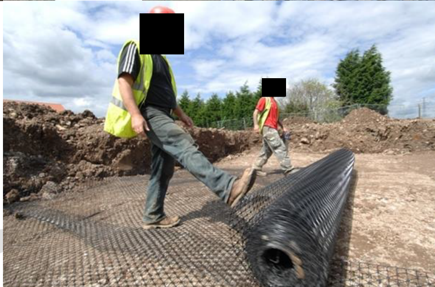
Examples of geogrid being laid to add additional strength to access roads
