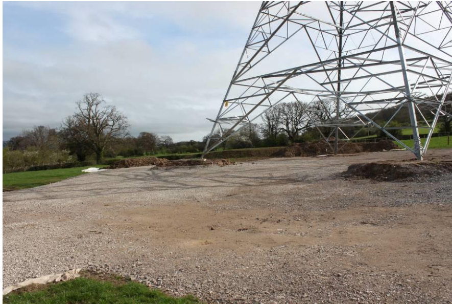
Typical working area
