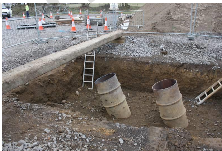
Typical excavation area for a pile cap (multiple piles per leg)
