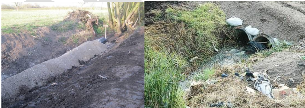
Examples of shallow culvert crossings
