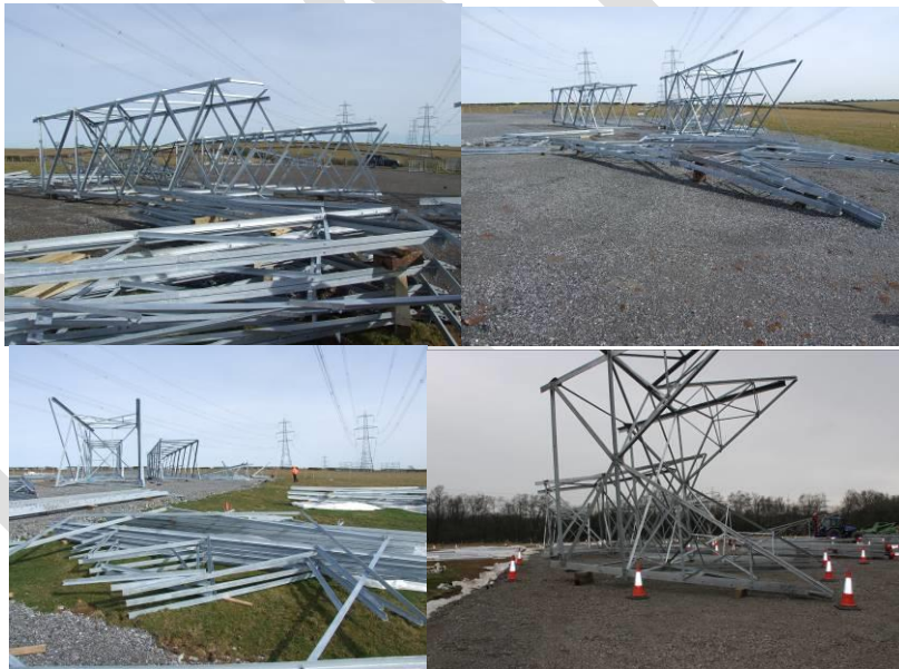
Typical layout of steelwork in preparation for erection
