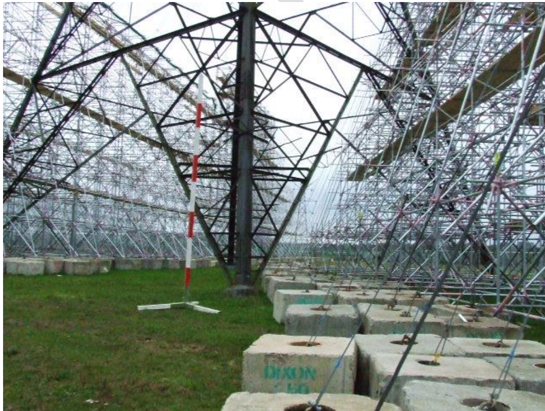
Kentledge blocks placed at the base of the scaffold.
