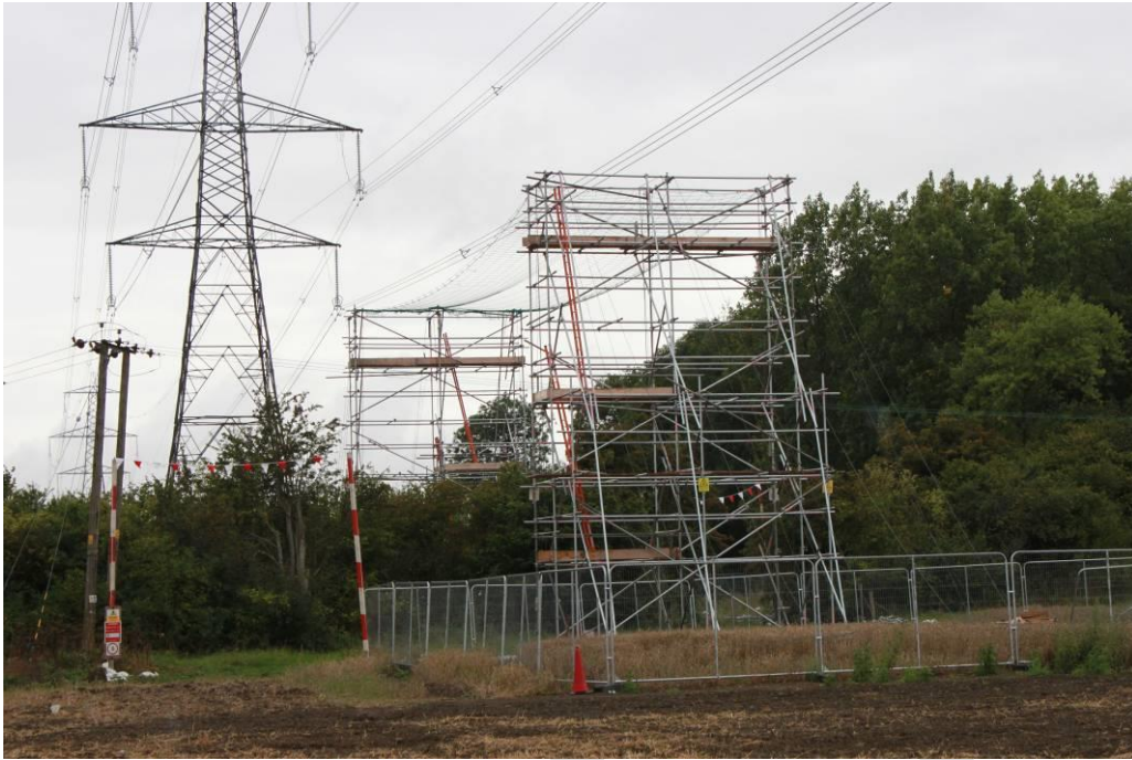
Scaffolding protecting an 11kV pole line
