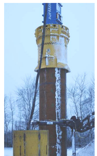
Figure 1 Pile crane and gripper (left) with pile hammer (right)
