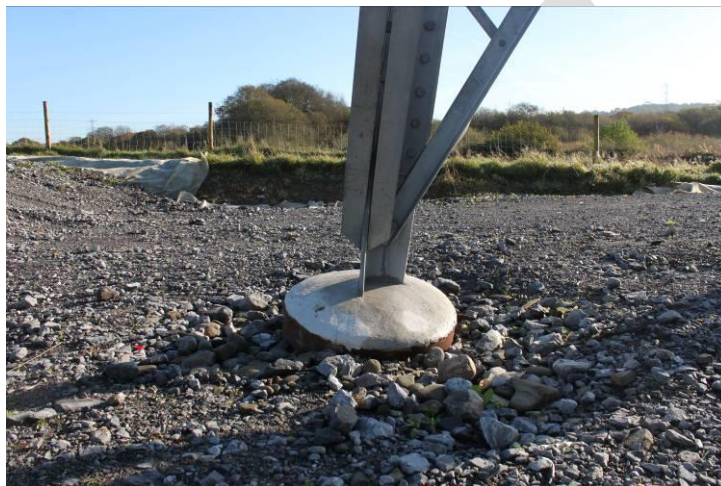
Finished piled leg on a typical line pylon with single tube (not pile cap).
