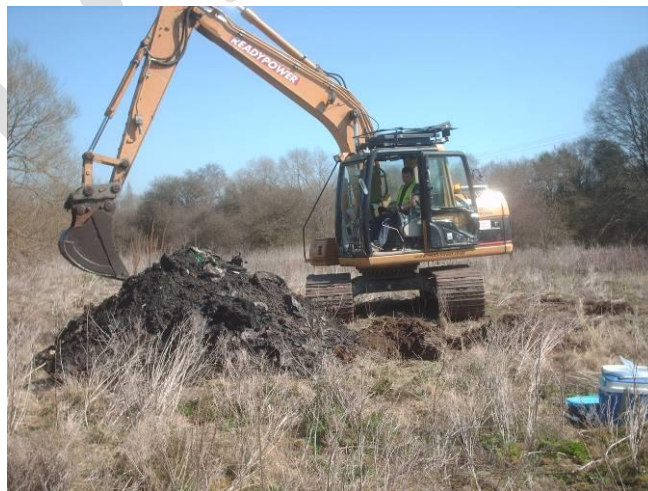
Trial hole excavation
