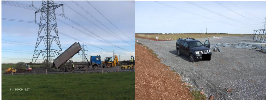
Access road and stone pad being installed
