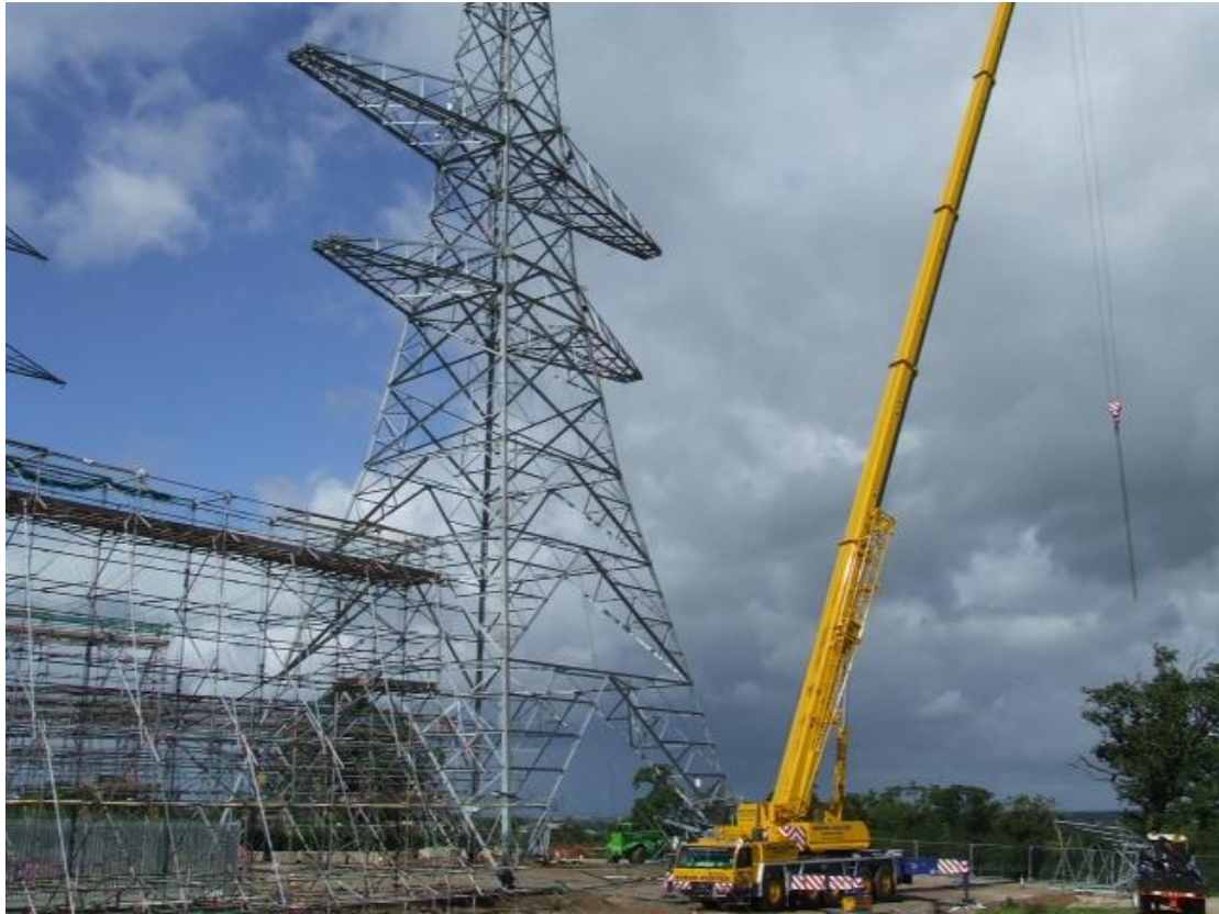
Crane positioned close to the pylon base
