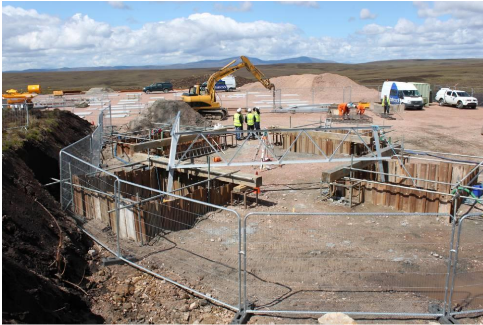
Typical Layout of a pad and chimney foundation (4 deep excavations) and a stub setting template being assembled
