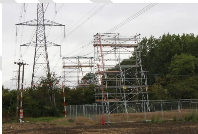
Scaffolding protecting an 11kV pole line
